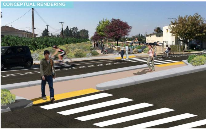
Figure 8-7: Road rebalancing on Gilbert Street would improve the crossing for trail users by reducing the number of lanes of traffic and providing a refuge median. The sectons below show the existing and proposed section view of Gilbert Street at the PE ROW Trail mid-block crossing.
