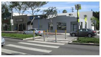
A midblock crossing in West Hollywood, CA features a high-visibility crosswalks, bollards, and flashing beacons for a safe, convenient walking environment
