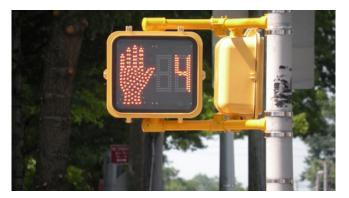
Pedestrian countdown signals provide timing information to pedestrians crossing the street and communicate pedestrian right of way to drivers
