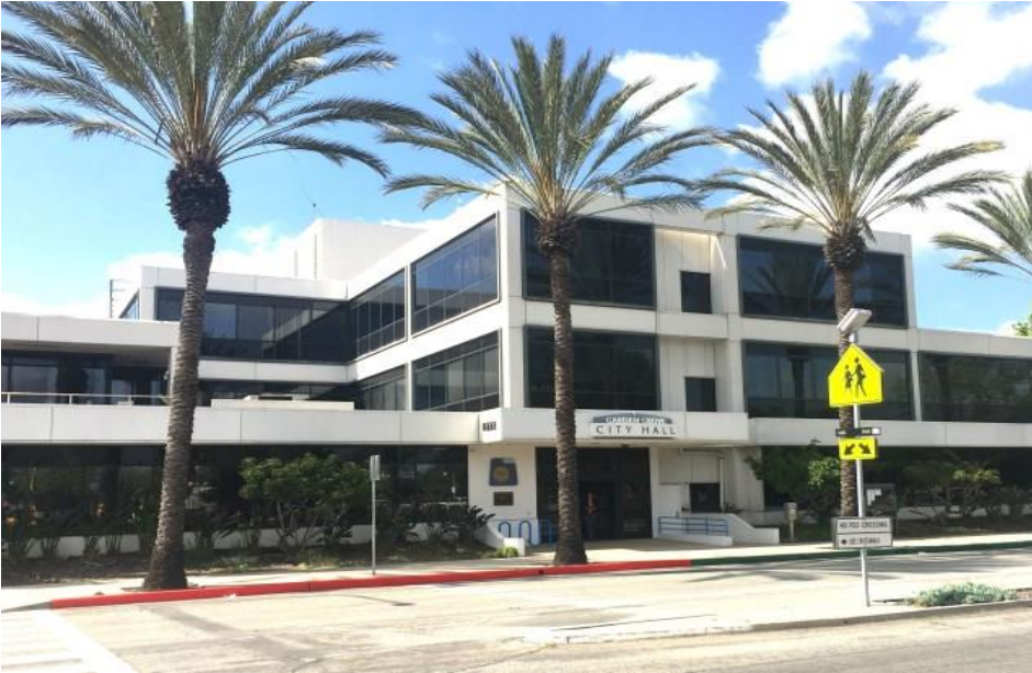
Garden Grove City Hall (Orange County Tribune photo)
